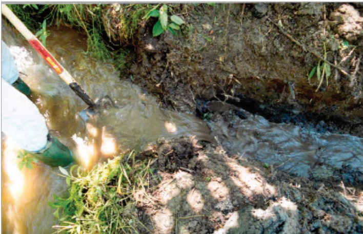
Figure 4.15c. Diversion trench August 2000.
