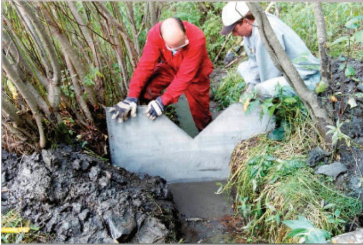
Figure 4.15d. Weir plate installation august 2000.
