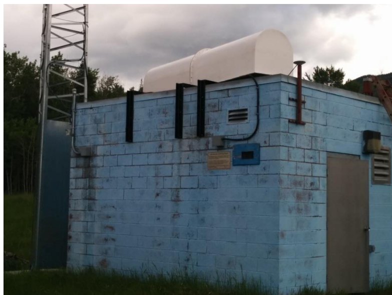
Figure 4. LiSAmobile system at the Bellevue pump house station.
