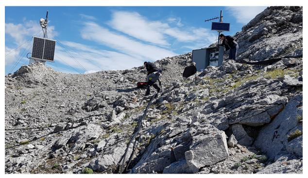
Figure 5. AGS field crew dismantling the borehole hub and conduit lines leading to multiple monitoring-equipment locations.
