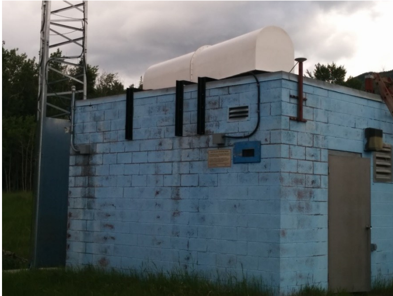
Figure 5. LiSAmobile system at the Bellevue pump house station.
