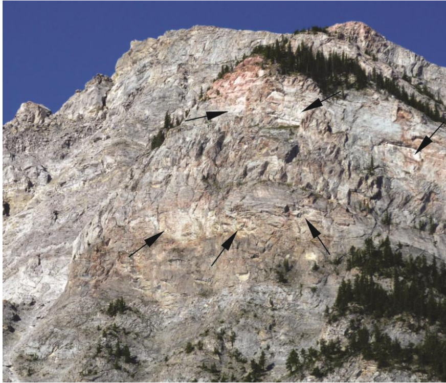
Figure 12: View towards the West of the main cliff showing fresh outcrops suggesting evidences of recent shallow block fall.
