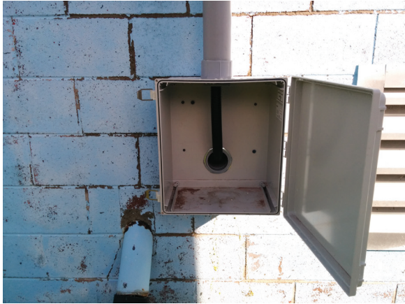
Figure 4. Installed 3" conduit pipe, weather box (left), and weather head (right) located at Bellevue pump house. Location of the LiSAmobile system.
