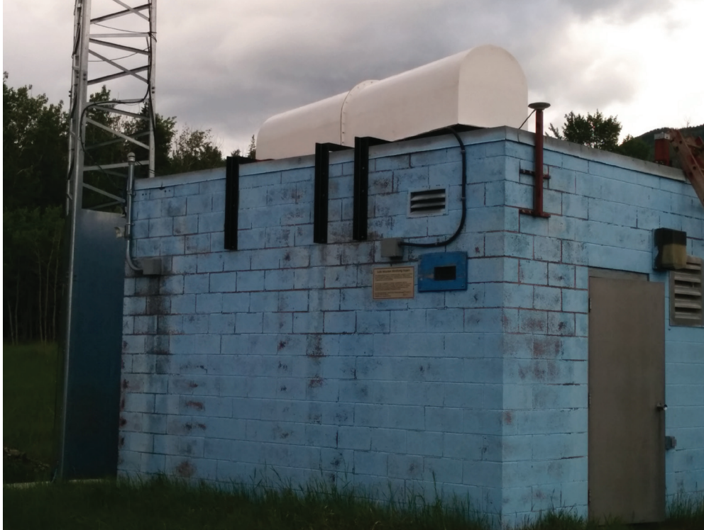
Figure 11. LiSAmobile system at the Bellevue pump house station.
