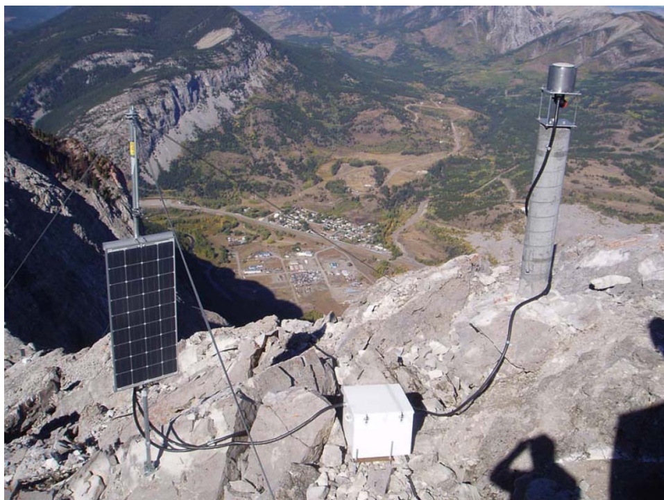
Figure 6. Typical differential GPS installation on Turtle Mountain, showing concrete pillar with Novatel antenna (right), battery box (centre) and solar panel (left). Enclosure hidden behind solar panel. Photo: G. Bjorgan, McElhanney Consulting Services Ltd.
