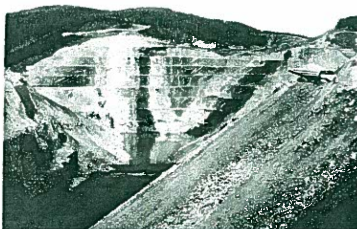
Figure 23. Anticline/syncline pair in CD Pit, with thickened Jewel Seam.
