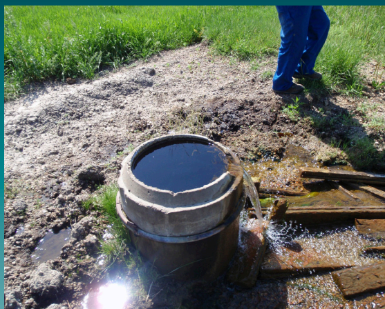
Flowing well in the central ECC encountered during sampling. Some wells, like this one, do not require us to connect our sampling equipment to the water well's plumbing system. The natural groundwater in the area has raised the water level above the top of the casing.
