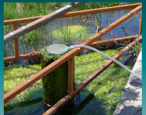
Groundwater discharge from a flowing well in the central portion of the ECC. The well water has risen above the top of the casing, forming a pond adjacent to the well.
