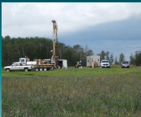
Drill site near Wetaskiwin, Alberta. A water-well rig completed all of the drilling for the ECC drilling program. Alberta Environment and AGS staff described all of the core on site and boxed the core for additional examination and analysis.
