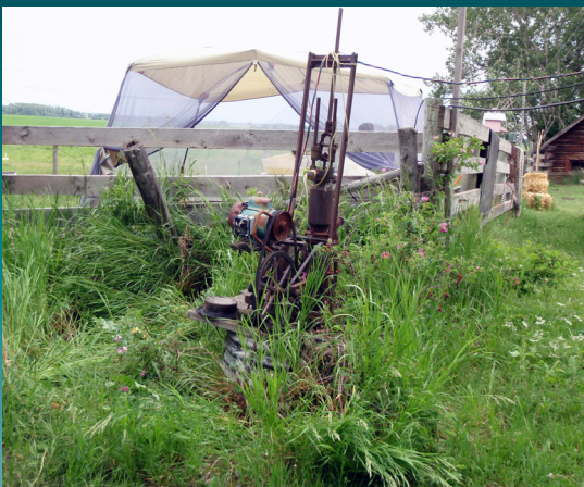
Creative water-well construction. Wells we sampled in the ECC came in all shapes and sizes. In this case, the well owner constructed the pump with parts on hand.
