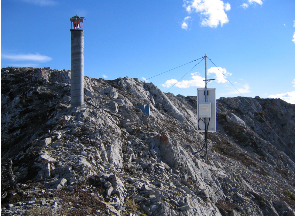
Figure 17. Combination theodolite prism and GPS antenna mounted on a concrete pillar near South Peak of Turtle Mountain. The prism is shown with an orange targeting guide; the oblate spheroid on top of the assembly is a GPS antenna.
