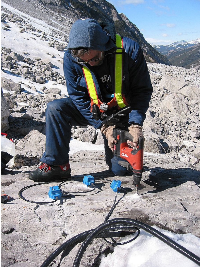
Figure 30. Installation of three-component geophones on Turtle Mountain.
