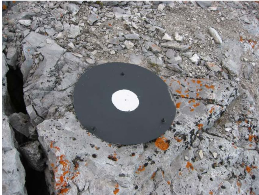
Figure 52. Photogrammetric target installed on Turtle Mountain in 1982 and repainted during the summer of 2005.
